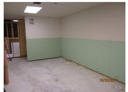
Below: Progress continues on the interior of the multipurpose building. Sheetrock is now installed in the restrooms. The leaves are beautiful and colorful, instead of the burned look.
